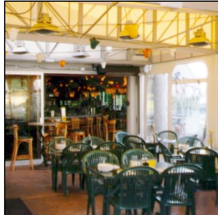
Zone controlled 3KW electric HotZone™ spot heaters warming the uninsulated restaurant at a golf course.
